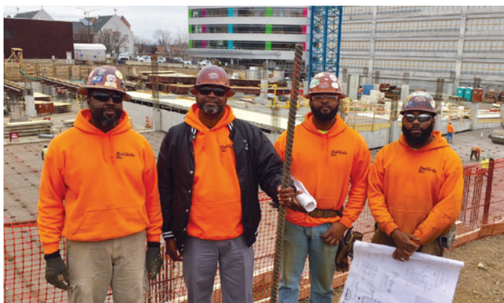
Larry Packer, Chris Packer, LeDon Packer and Mike Bell, Jr. all from Rod-Techs and all family members working on the Northern Avenue garage.
